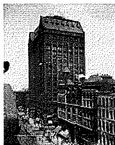
The Masonic Temple Chicago's Great Skyscraper (265ft) Randolph and State Street 1900
